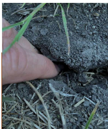
Clay soils from Red River Valley showing lack of moisture as it starts to crack.
